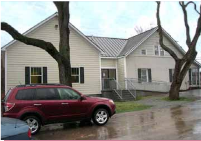
HospiceCare's Lewisburg Office, above, has moved to a newly renovated building at 223 Maplewood Avenue across the street from the Greenbrier Valley Medical Center. We believe the new facility will offer greater visibility for our local programs and services. Below, the new entry sign at the Charleston Main office. At right, the street sign at the corner of Kanawha Boulevard and 2nd Avenue at Patrick Street. Below right, a large crowd gathered for the formal ribbon cutting ceremony.
